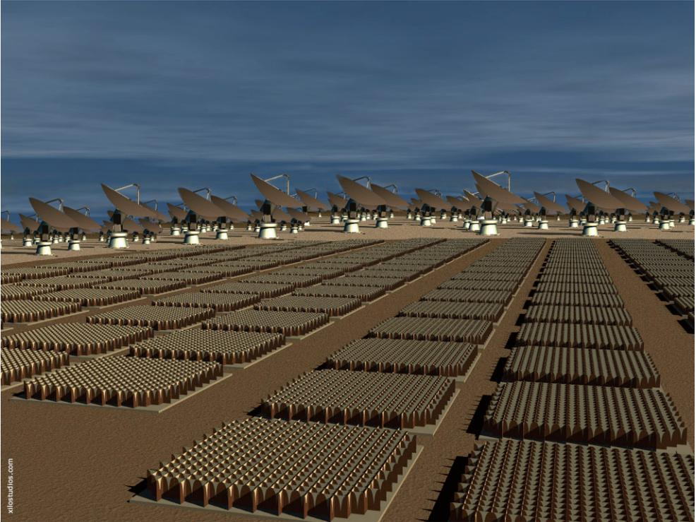
Figure 1.: *An artist's conception of a SKA station. The Aperture-Plane Phased-Array occupies a large area, with many small receiving elements viewing the sky directly. This technology provides a very large field of view, and digital technology permits a large number of synthesised beams to fully sample the field of view with high spatial resolution. [10]*
