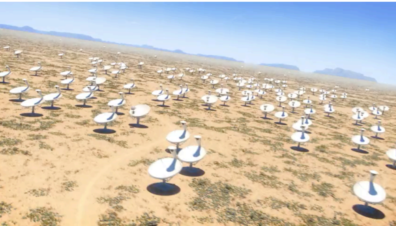
SKA-Mid : 350 MHz - >20 \text{ GHz} 200 parabolas, South Africa
